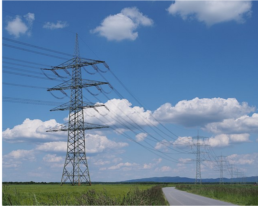
Figure 1.1: Overhead electric transmission lines. Image courtesy of Kreuzschnabel/Wikimedia Commons [44].
