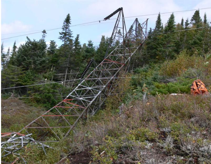
Figure 1.1: Power line failure due to WIV in Ontario
