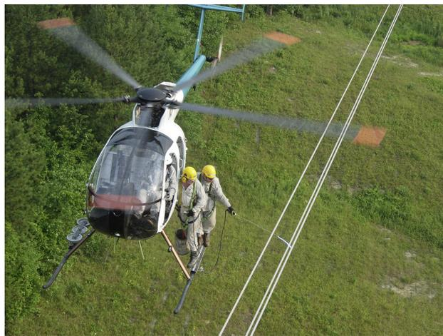
Figure 1.8: A helicopter-assisted repair of a power line
