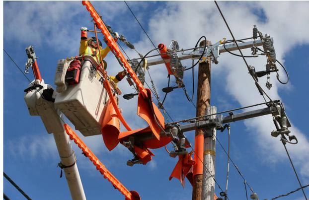
Figure 1.7: Manned repair of a power line.
